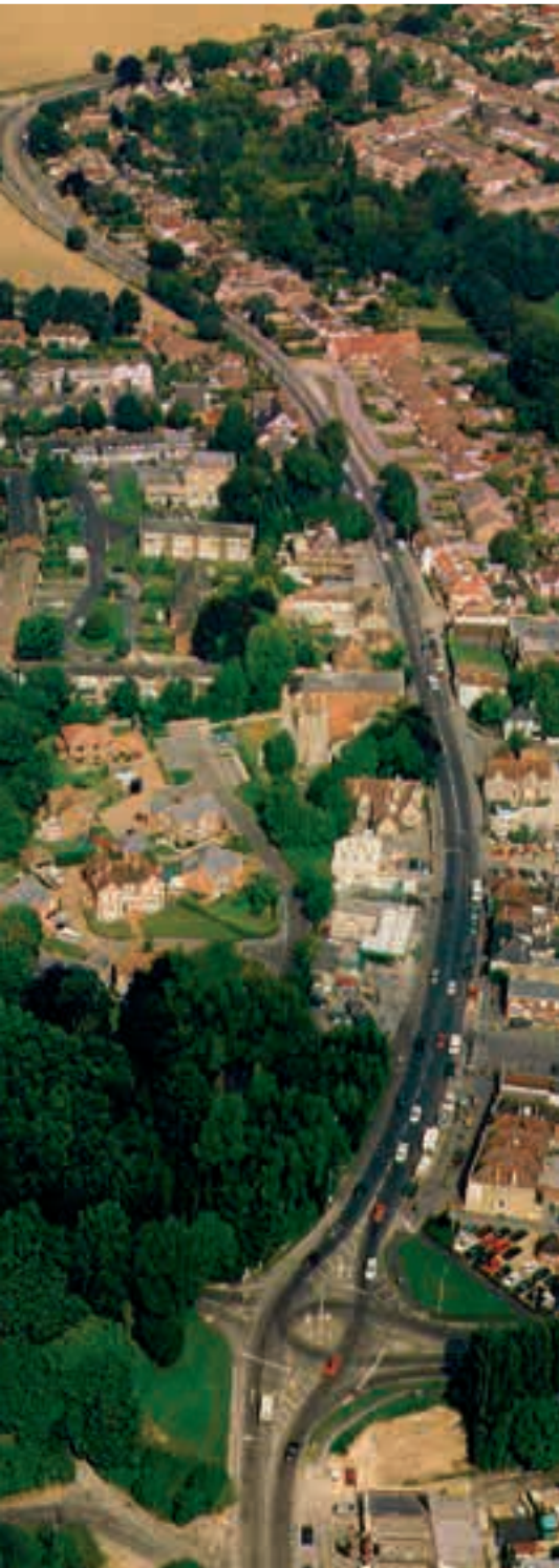
A3 Bus Priority Project - Purbrook Village
