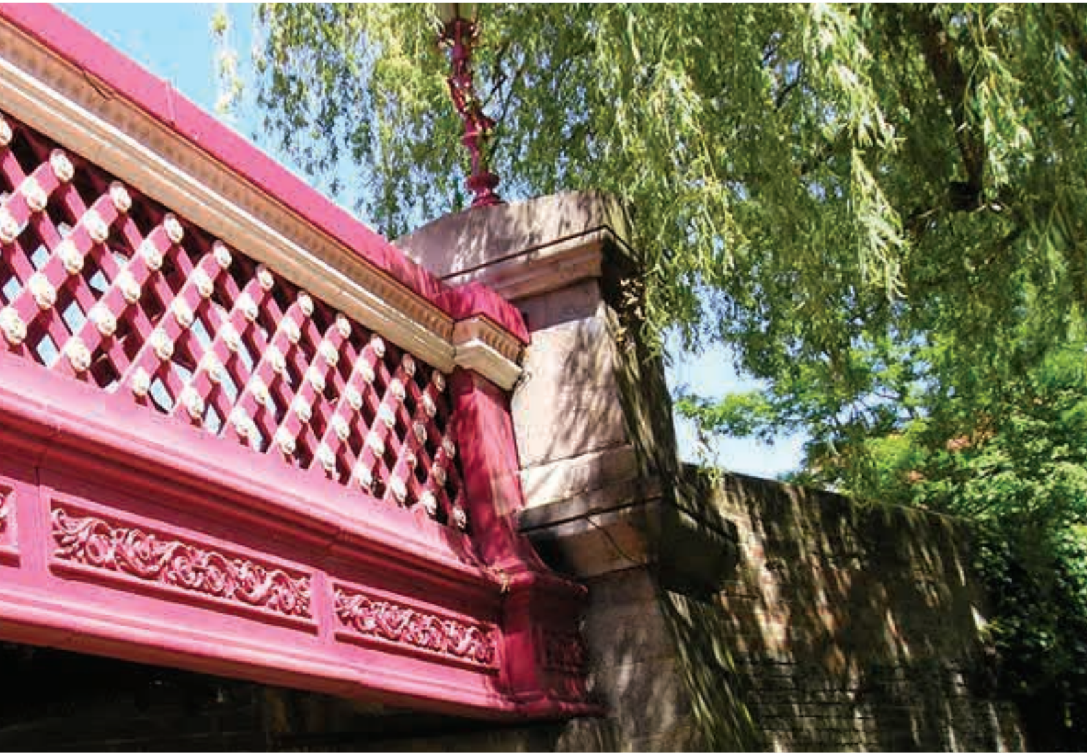
Barnespool Bridge - Eton
